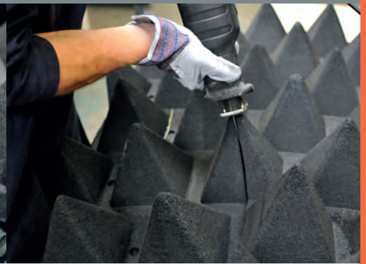
Easy to adapt to site specific requirements with the use of a reciprocating saw.
